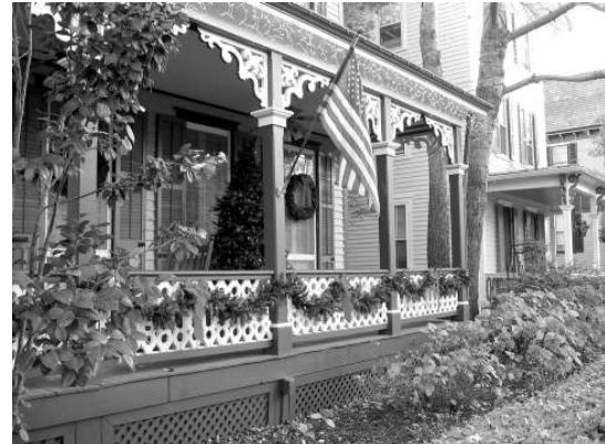
The Henry Sawyer Inn at the corner of Columbia Ave. and Franklin St.
